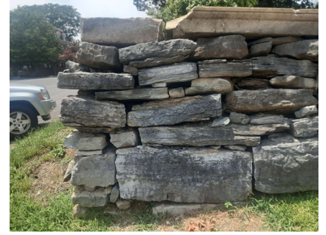
3 1 Example of existing stone wall N/A
