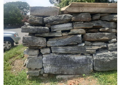
3 Example of existing stone wall 1 N/A
