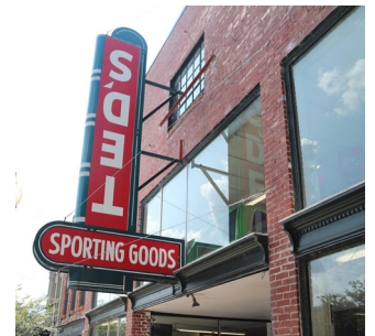
TED'S SPORTING GOODS SIGN RESTORATION AND ILLUMINATION
