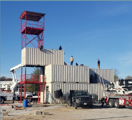
Fire Department Training Center Construction
