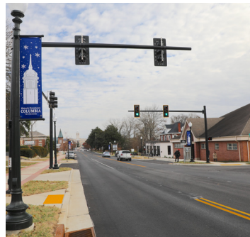
WEST 7TH STREET STREET SCAPE CONSTRUCTION
