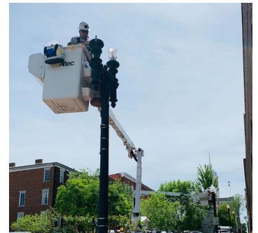
LED STREET LIGHT CONVERSIONS CONSTRUCTION
