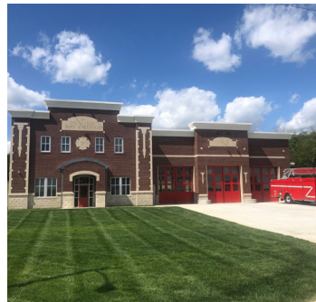
FIRE STATION NO. 3 COMPLETED
