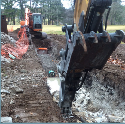
Wastewater system-wide improvements
