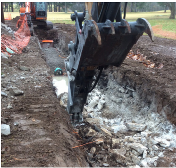
WASTEWATER SYSTEM REHAB CONSTRUCTION
