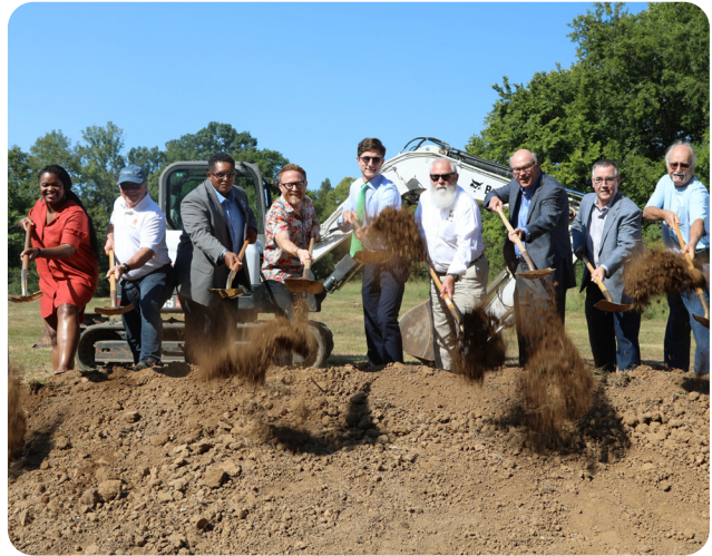
Groundbreaking for new wastewater treatment project, the largest project in City history totaling $97 million for construction.
