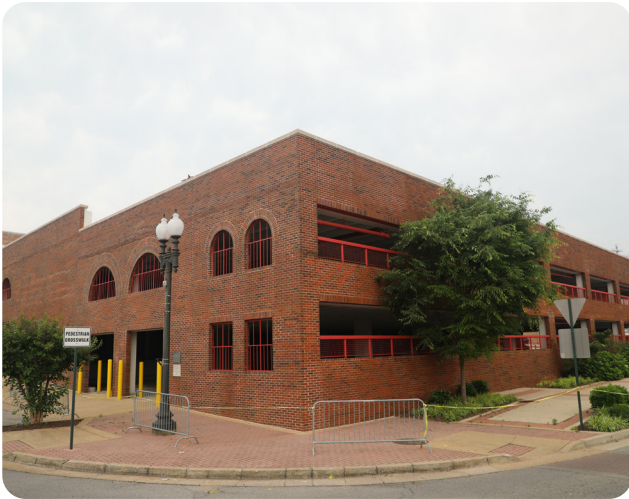
Garage renovations in 2024 totaled nearly $900,000, repairing brick and water damage through the structure.
