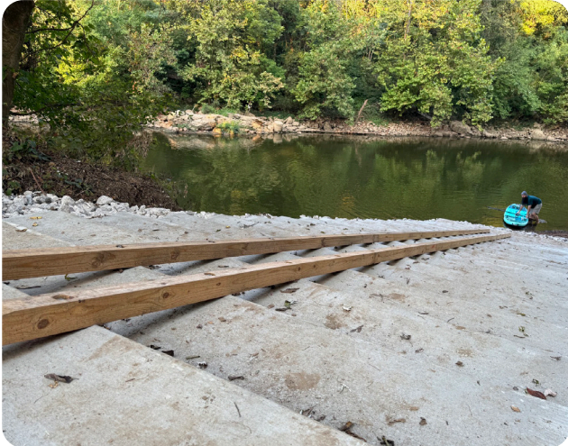
Canoe launch construction using tourism grant
