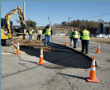
Burt Dr and Nashville Hwy intersection improvements
