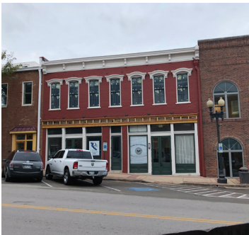
JACK-N-JILL BUILDING CONSTRUCTION
