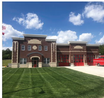
FIRE STATION NO. 3 CONSTRUCTION
