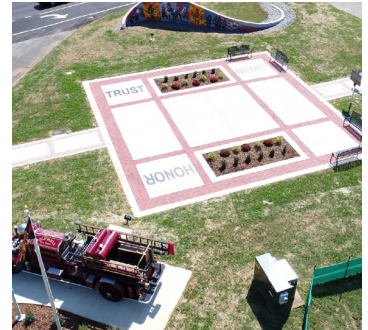
FIREFIGHTERS PARK CONSTRUCTION OF PHASE I
