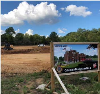
COLUMBIA WORKS PROJECTS LOCAL, HIGH-IMPACT INFRASTRUCTURE IMPROVEMENTS
