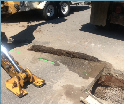
Wastewater removes root mass from mainline at Riverwalk Park
