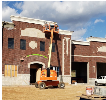
NEW FIRE STATION NO. 3 CONSTRUCTION
