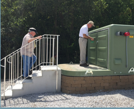
Pump Station Replacement
