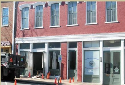
Jack-N-Jill Building Project-Exterior Construction Phase
