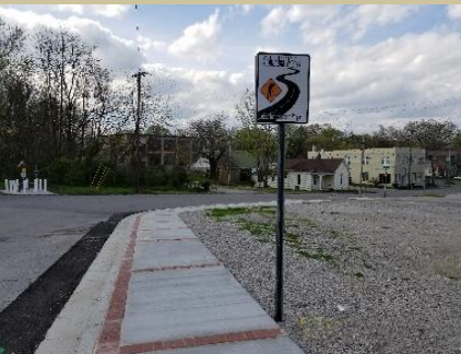
Columbia Works - Depot St. Sidewalk Improvements/ADA Crosswalks
