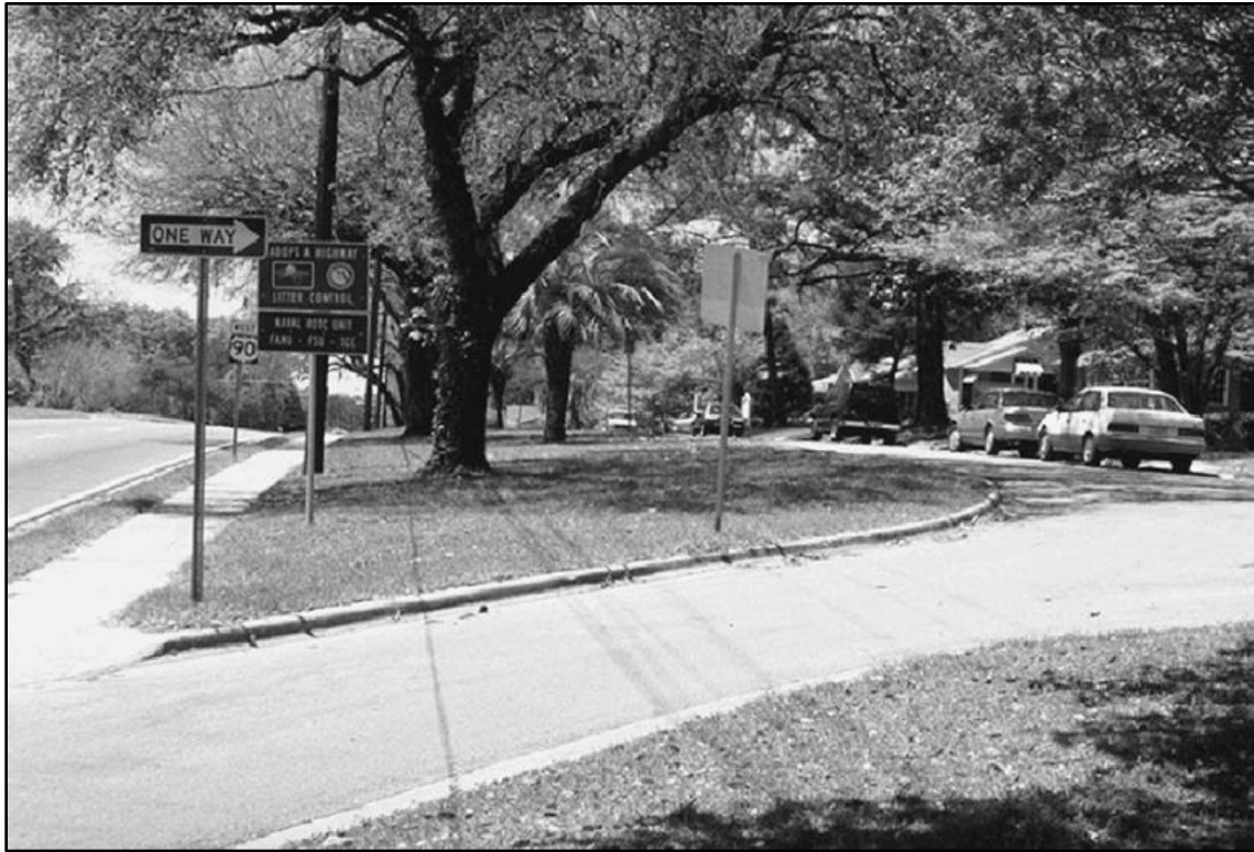
Figure 12: Frontage roads in residential or light office areas can work well where they are one way and begin and end between major crossroads.
